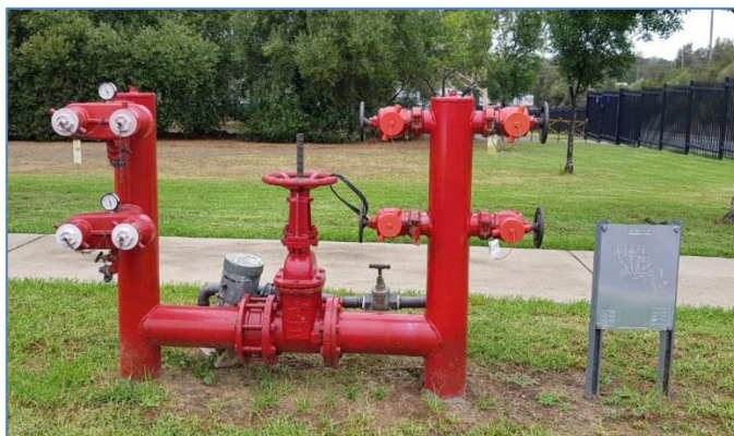
F. Existing fire hydrant booster assembly and block plan
